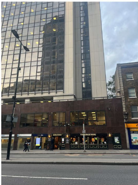
Figure 15 - View of existing Public House on Wormwood Street facing north.
